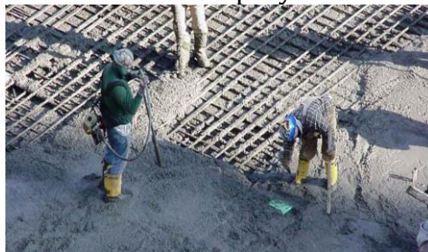
Gambar 2.1 Beton Site In Cast
