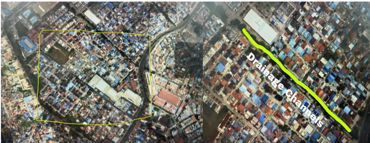
Figure 1. Location survey of the drainage
