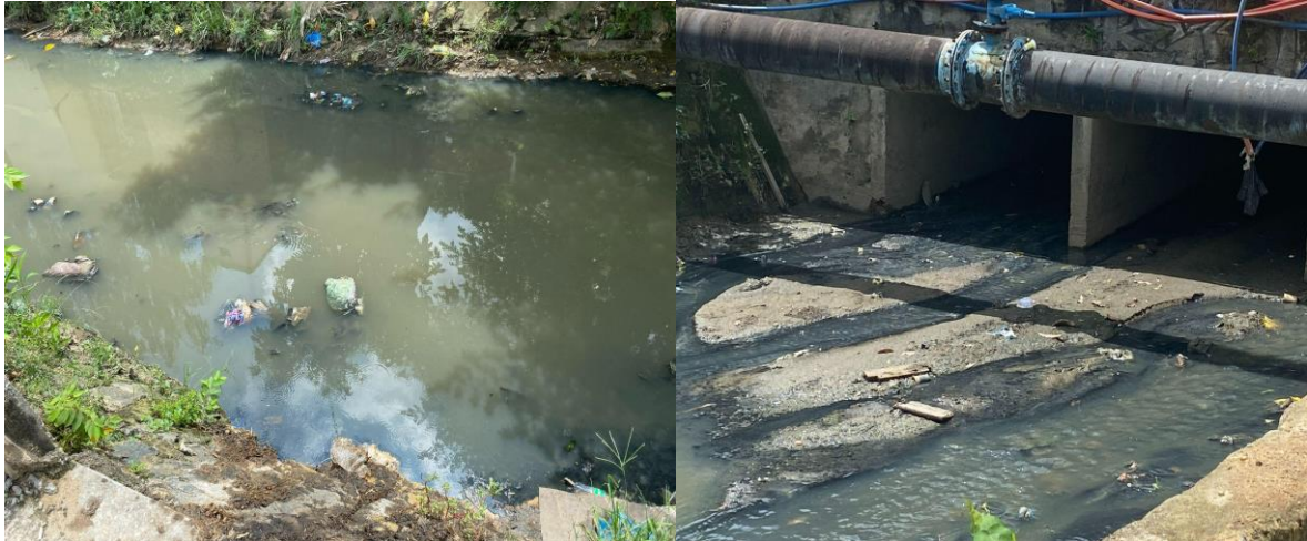
Figure 2 Nagoya Drainage conditions with garbage and Sedimentation
