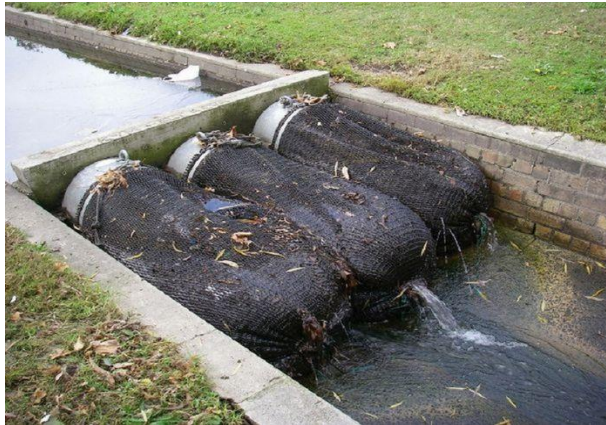
Figure 4. Net trap to increase drainage water flow and Prototype sediment traps
