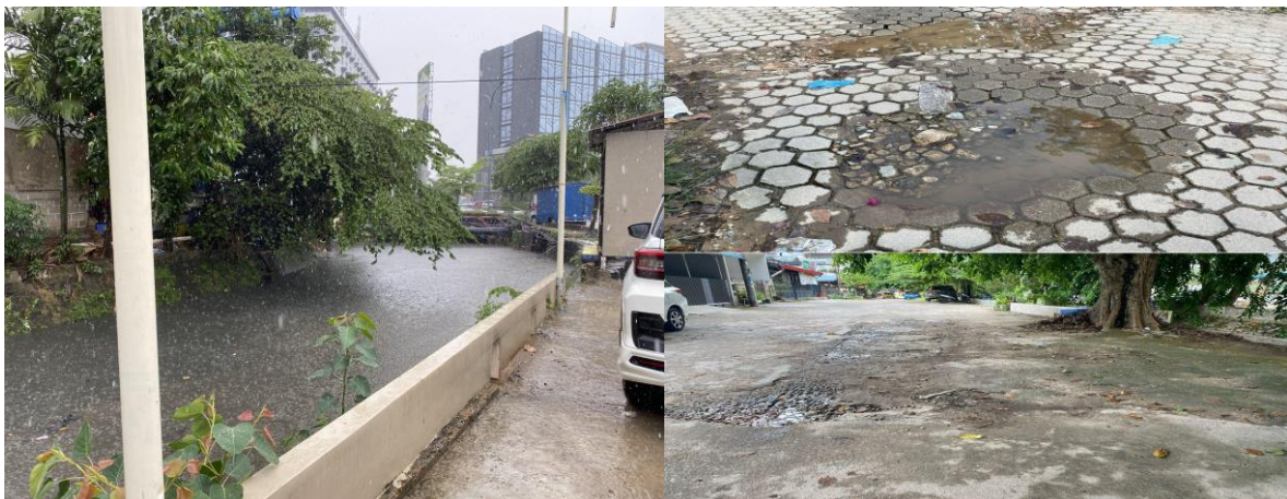
Figure 3. Drainage and submerged by flood
