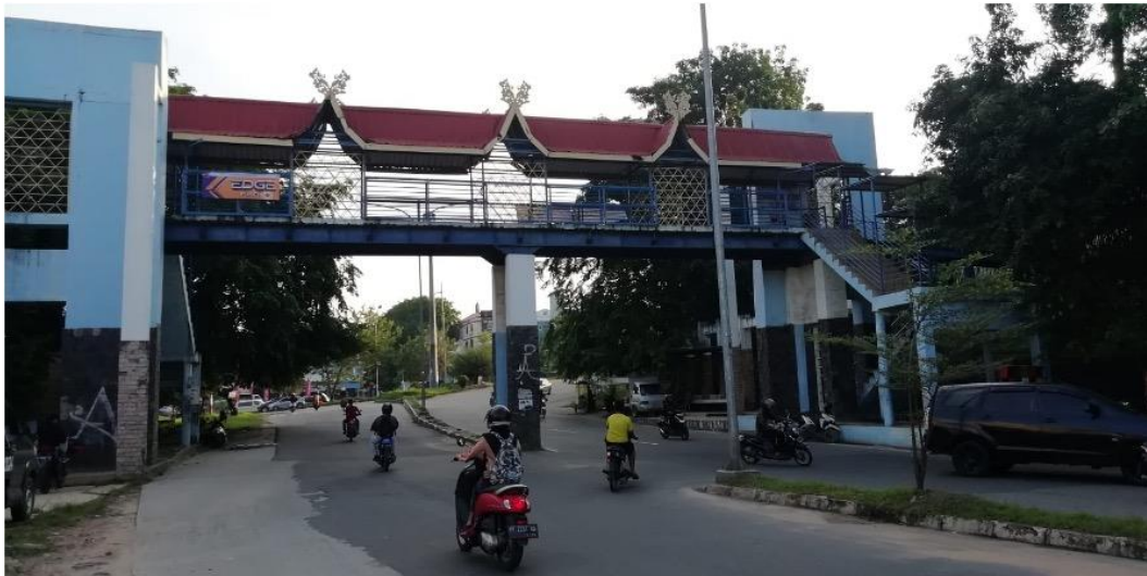
Figure 1. The overhead crossing bridge
