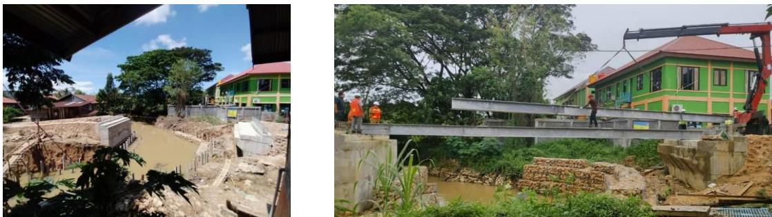
Figure 3. Kanaan Bridge under construction work (Source: Google, 2023)
