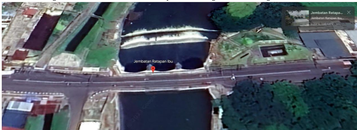
Figure 2. Location Of Ratapan Ibu Bridge, Payakumbuh, Padang (Source: Google Earth)
