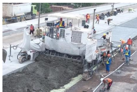
Figure 3. Implementation of Rigid Pavement with Concrete Pavers Source: author documentation
