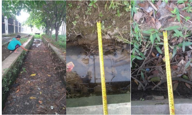
picture 1.3 Measurement of Drainage Diameter and Observation of Drainage conditions
