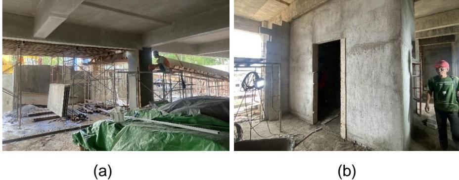
Gambar 1. (a) Pekerjaan *Skimcoat* Beton Lantai Semi *Basement*. (b) Plaster Dinding Lantai 4.
