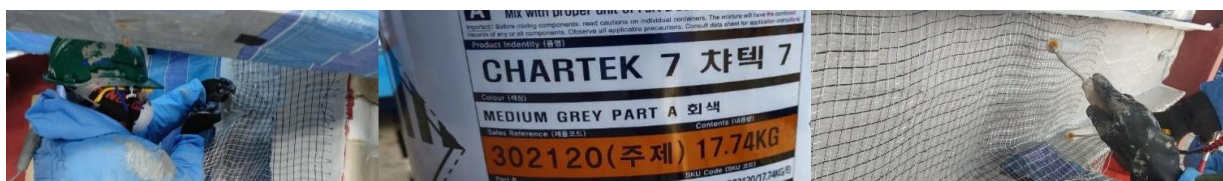
Fig 5. Intumescent fireproofing application with Chartek 7
