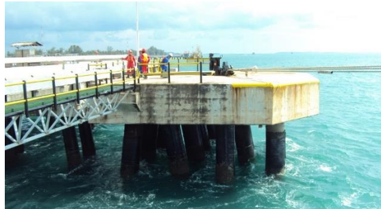
Gambar 3.1 Mooring Dolphin 6, Jetty 7 PT. Pertamina Tanjung Uban (Tampak Depan)
