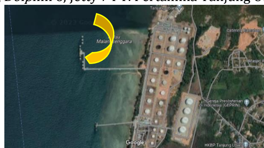
Gambar 3.2 Area Mooring Dolphin 6, Jetty 7 PT. Pertamina Tanjung Uban (Google View)
