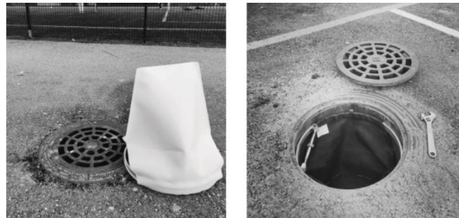
Figure 10. Sediment traps on manhole cover
