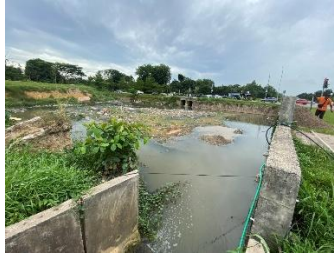
Figure 6. Sediment build on drainage channels, Batam Kota Sub – District, Source : Real Time Observation
