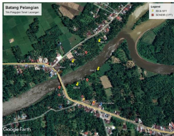
Fig 2. Soil investigation (CPT and SPT) locations Source: Project report
