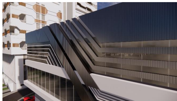
Figure 8. ACP and Glass Material on Facade Source: Author, 2023
