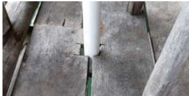
Figure 13. Sink Channel that Flows Directly into the Sea
