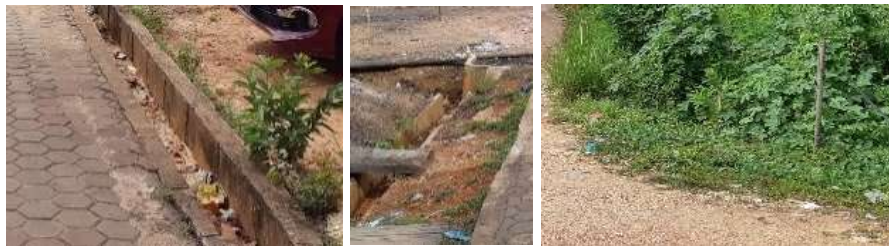
Figure 10. Small Plastic Wastes that are Disposed of Improperly Source: Authors, 2021
