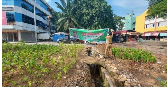
Installation of a warning banner not to throw trash indiscriminately
